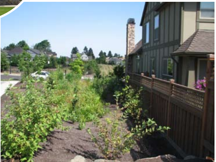
In Wilsonville’s Villebois community, use of water gardens, left, and rain gardens, right, allow rainwater to soak into soil creating a slower delivery of cleaner water into nearby rivers and waterways. Porous street pavers also help filter large amounts of water.
